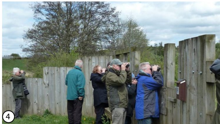
④ An open wildlife/bird hide made of chunky timber sleepers offering 'windows' at various heights to view the wetland cells whilst being a sculptural feature in keeping with the site design
