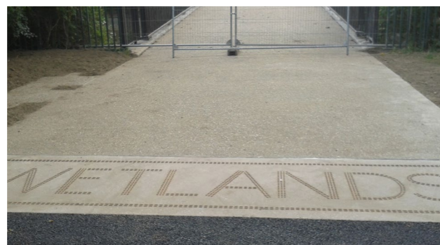
Paved surfaces Exposed aggregate concrete footpaths are durable and give a buff coloured finish
