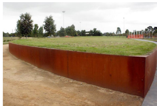
Main Entrance Feature Corten steel is a durable high quality material which can be used as a retaining wall
