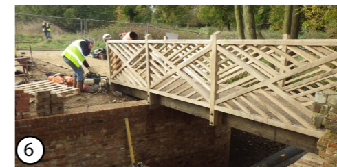
Example of a type of footbridge used in the borough
