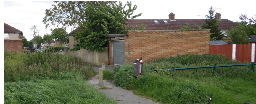
Existing view of eastern entrance No.2
