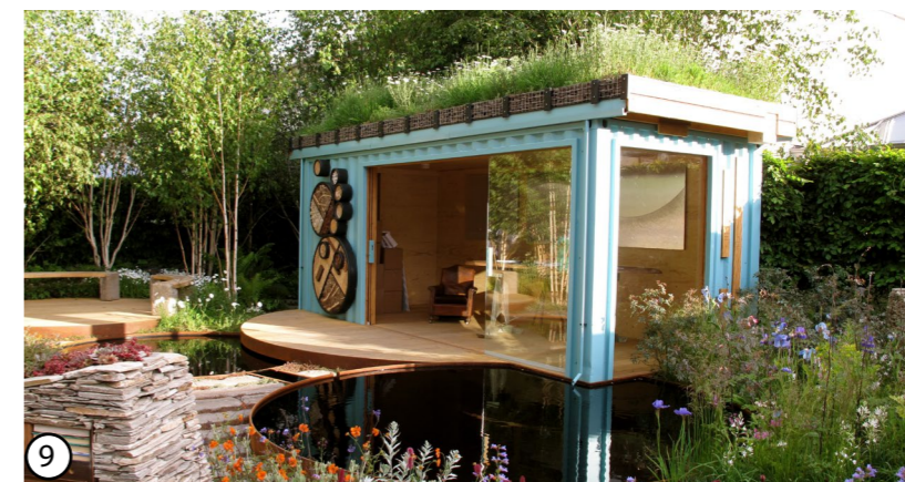
Example of a potential wetland community facility, a shipping container renovated with green roof
