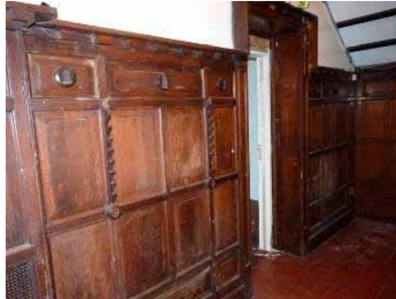
Figure 54 Back Hall showing south elevation
