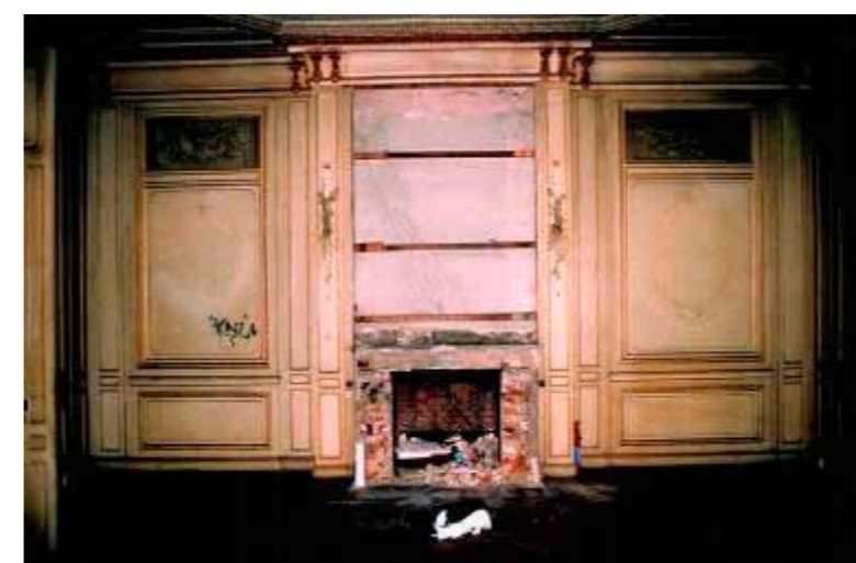
Figure 31 State of Drawing Room fireplace wall 1996
