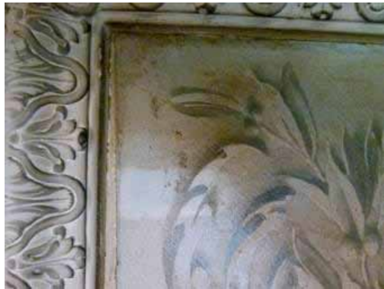
Figure 23 Drawing Room, cleaning trial to ceiling panel grisaille reveals subtle tones of original painting
