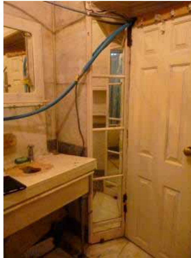
Figure 94 Bathroom, north east corner
