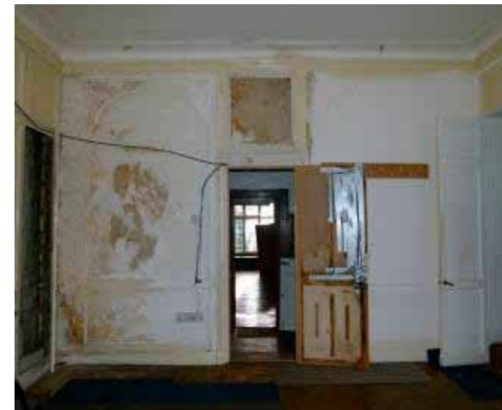
Figure 62 North East Bedroom, south elevation showing large area of wall affected by damp
