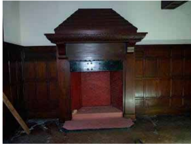
Figure 10 Living Hall, north elevation, fireplace
