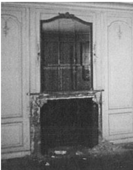
Figure 110 South West Bedroom, early photograph showing over-mantel mirror, the fire surround is missing
