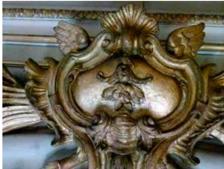
Figure 27 Drawing Room, showing surface cleaning to right side of moulding
