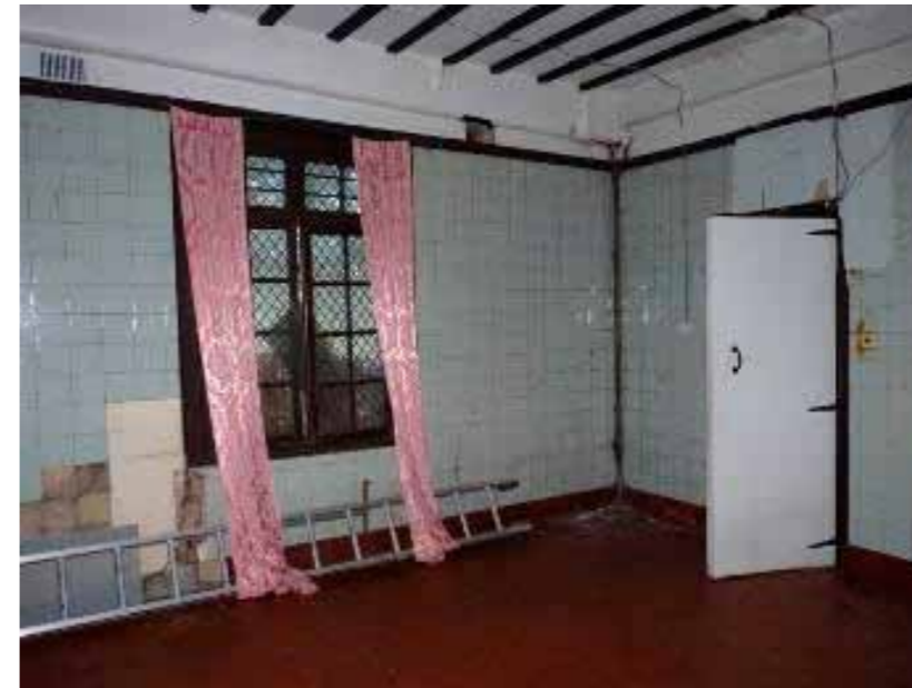
Figure 48 Kitchen south-east corner
