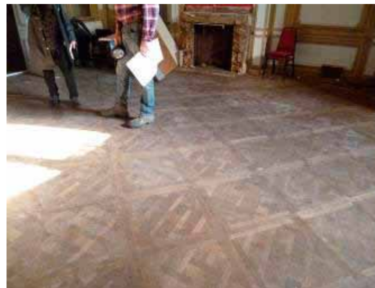
Figure 16 Drawing Room, parquet flooring
