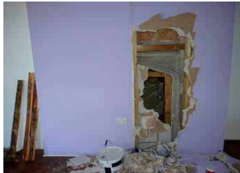
Figure 42 Dining Room, plasterboard removed to reveal original fireplace
