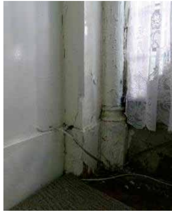
Figure 59 East end lobby, showing damage caused by damp conditions
