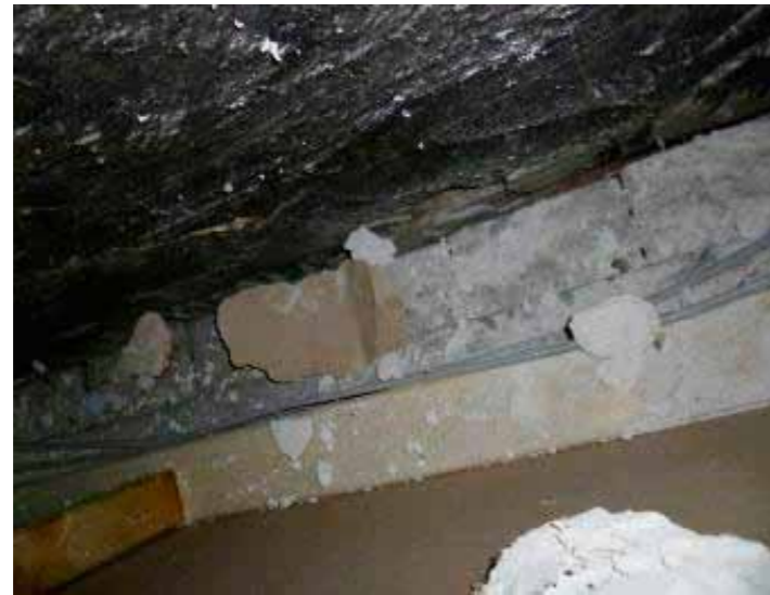
Figure 37 Dining Room, behind the plasterboard shows plaster walls and no panelling
