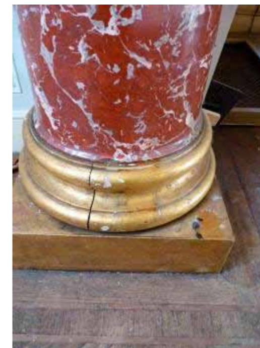
Figure 18 Drawing Room, south elevation, showing cleaning trial to scagliola columns base
