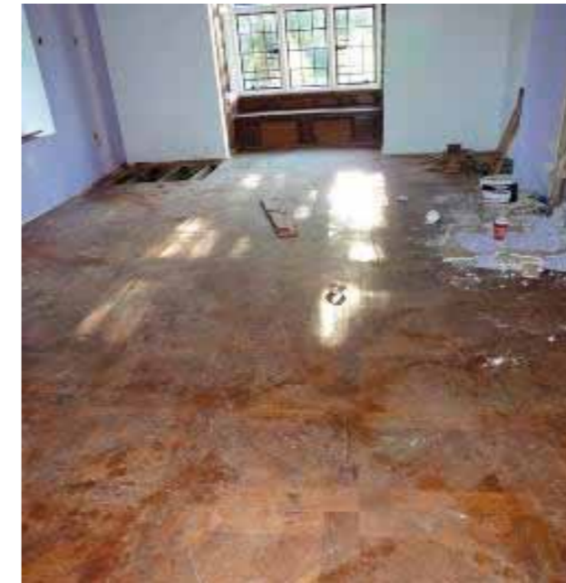
Figure 34 Dining Room, parquet flooring showing signs of wear and tear
