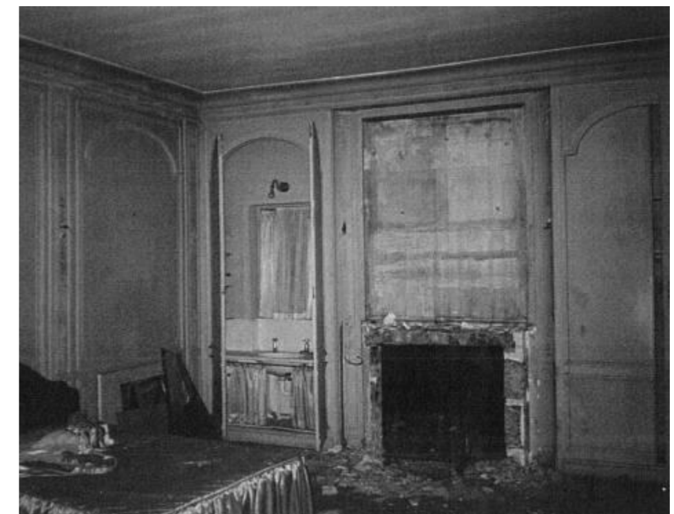
Figure 68 North East Bedroom, early image of room showing missing fire surround and over-mantel
