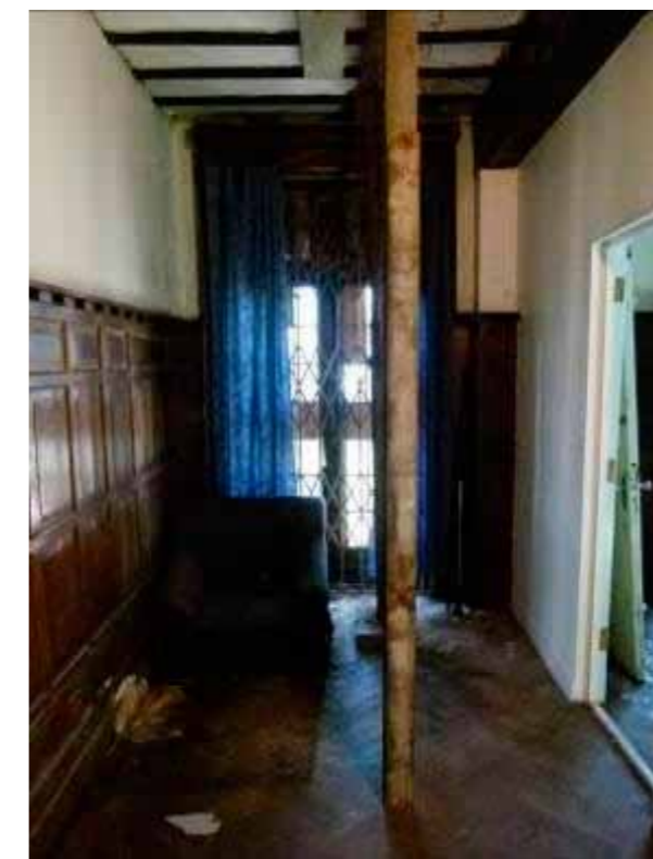
Figure 4 Entrance Hall showing new partition wall and area of rot to timber on lower left side
