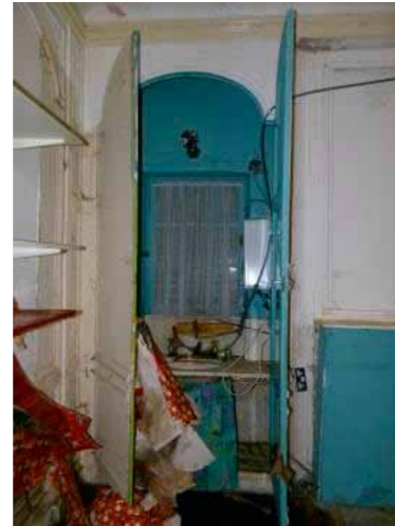
Figure 67 North East Bedroom, wash area with basin plumbed into cupboard
