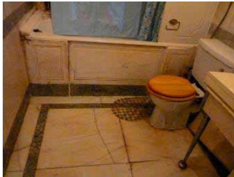
Figure 90 Bathroom, marble floor and bath surround showing cracks and staining
