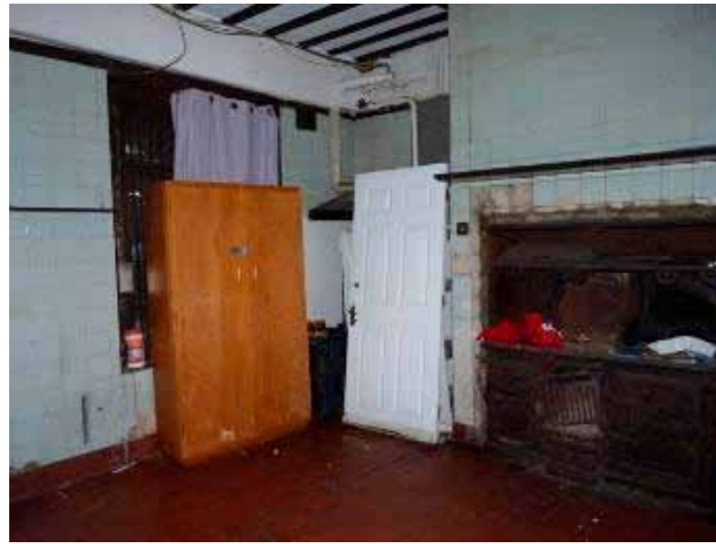
Figure 45 Kitchen north-west corner
