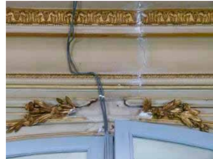
Figure 25 Drawing Room, detail of damage and loss to moulding over the doors
