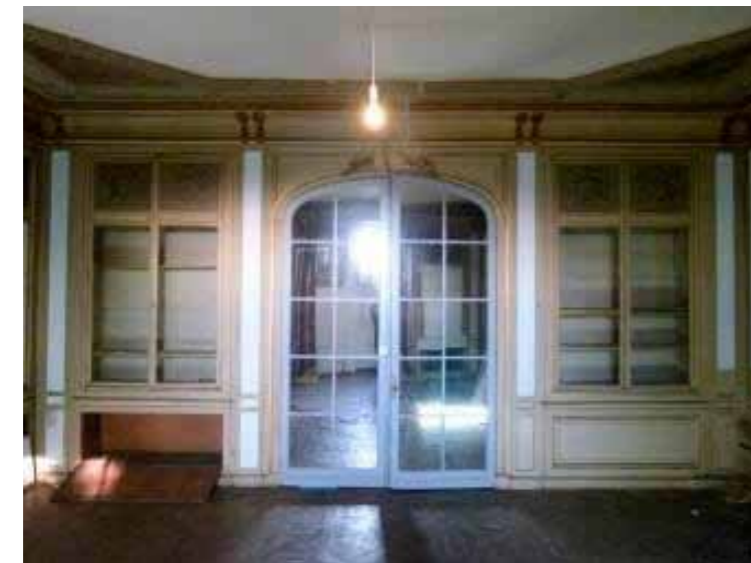
Figure 15 Drawing Room, north elevation, showing mirror backed double doors
