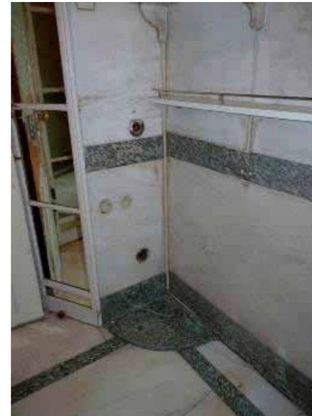
Figure 92 Bathroom, view of south east corner showing cracks and staining to marble
