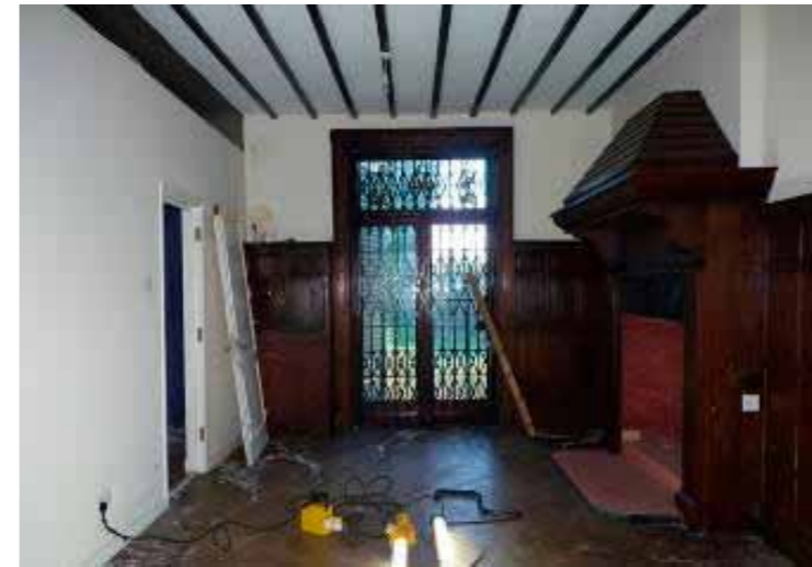
Figure 8 Living Hall, general view towards west elevation
